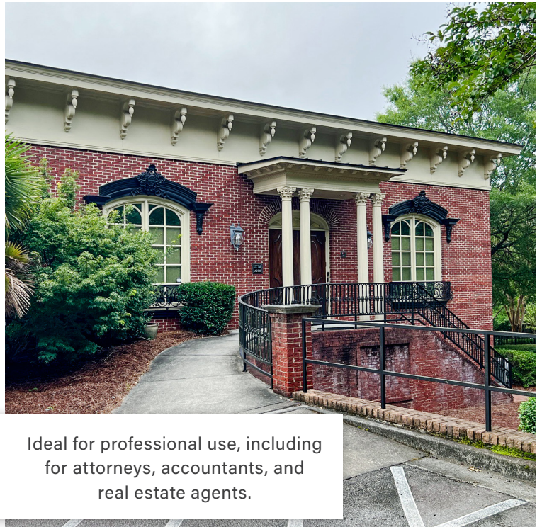
BUILDING 8450, STE 100 4,861 SF
